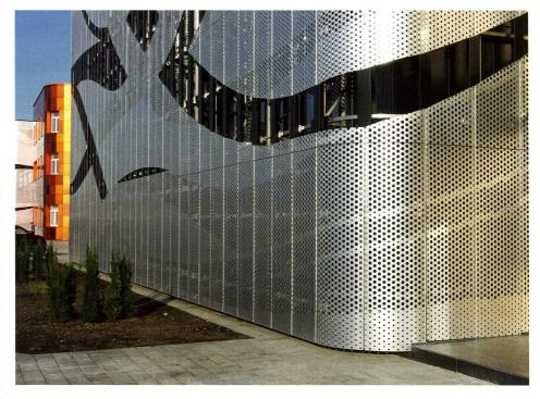
J73A UP coil anodized aluminium, natural anodized color, were used for the dynamic design. The 2.0 mm thick aluminium panels, perforated with hole diameters of 20, 25 and 37 mm, which were processed and installed by RannBuilding OOO, give the façade a certain lightness.
